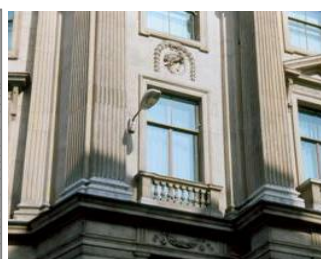
Street lights on buildings
