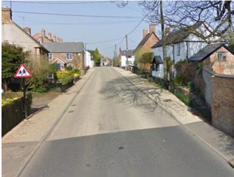
Whittlebury change of surface colour at village entrance
