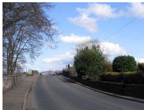
Clifton, hump back bridge after safety scheme
