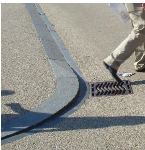
Changes to road and pavement design help
